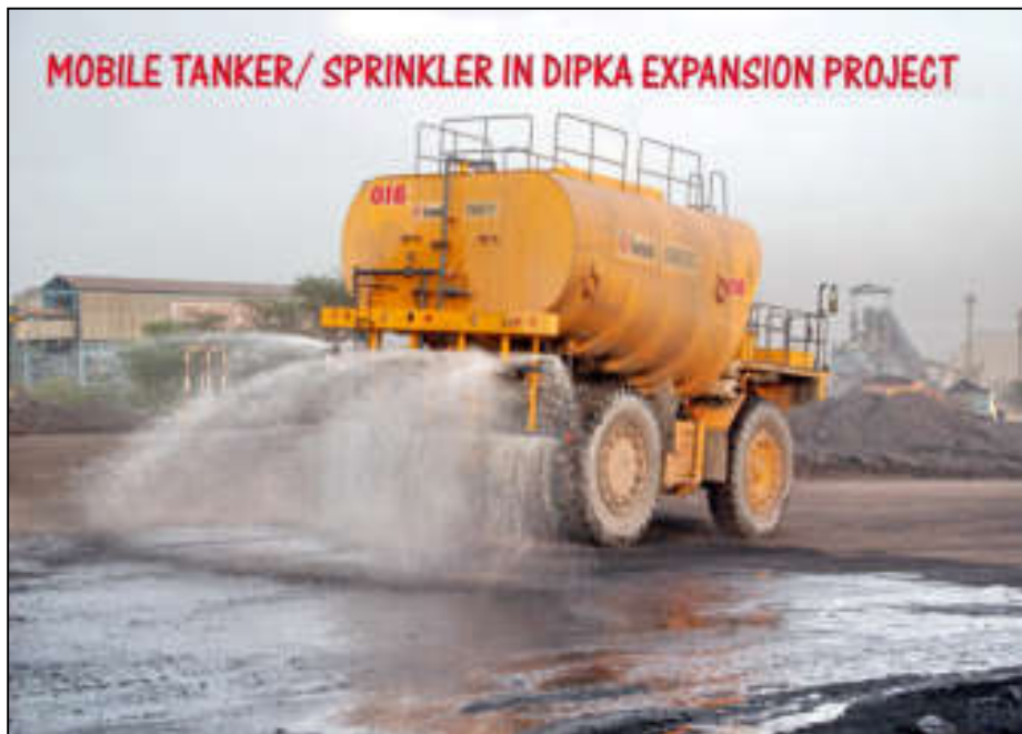
Fig-2: Mobile Water Sprinklers
